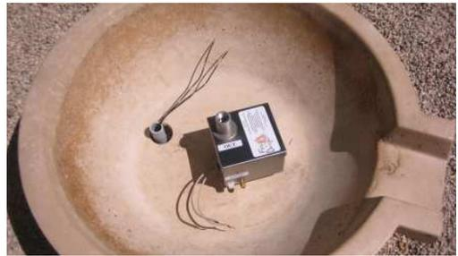
3. Electrical Connections. In the photo at right the wires protruding from the AWEIS has been connected to the two wires from the electrical conduit using appropriate sized wire nuts.
